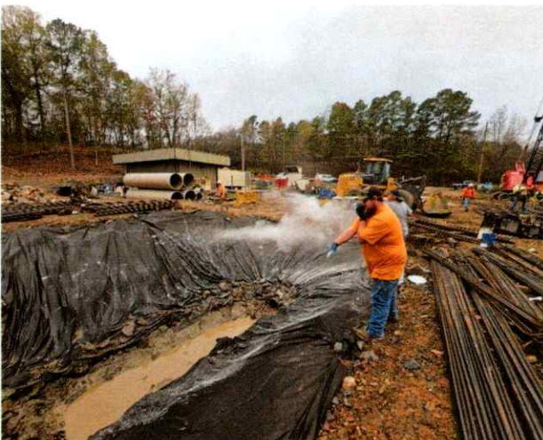
MH 1748 During Cleanup – 11/5/2024
