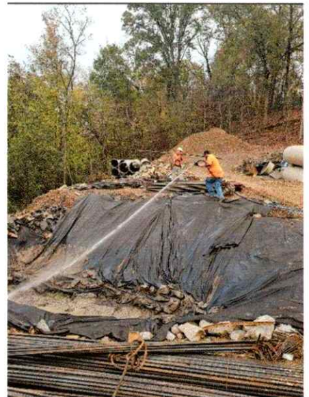
MH 1748 During Cleanup – 11/5/2024
