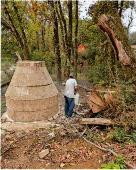
MH 1748 During Cleanup – 11/5/2024
