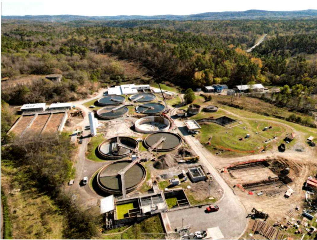
New Clarifier construction - Davidson Drive Wastewater Treatment Plant
