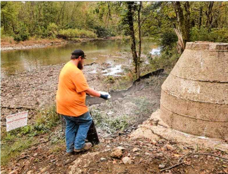
MH 1748 During Cleanup – 11/5/2024
