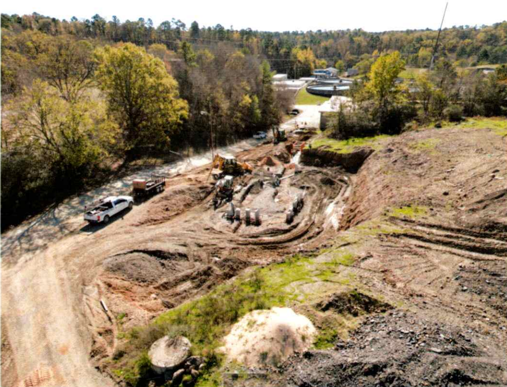
Emergency Generator Pad construction - Davidson Drive Wastewater Treatment Plant
