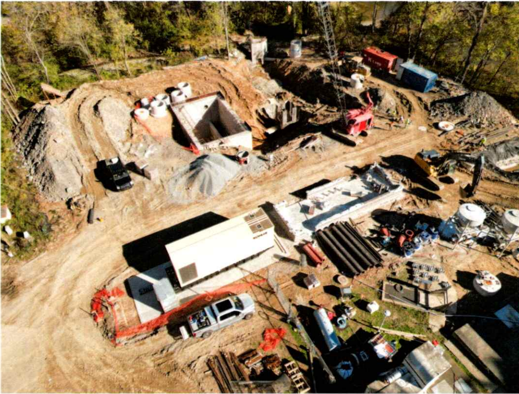
Gulpha Pp Station construction
